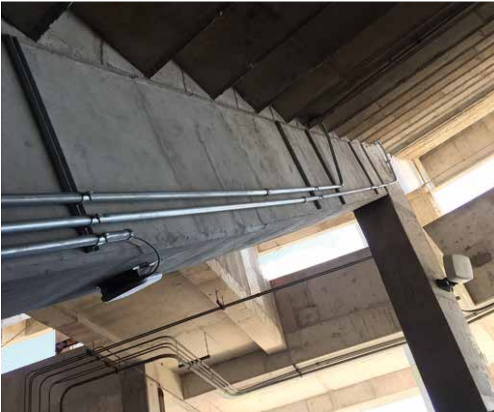
CONDUIT HEADS UPHILL TO UNDER-SEAT CORE DRILLS; AN EXPRESS PICKUP LANE AT A CONCESSION STAND; AND ONE OF FLORIDA'S HEISMAN HEROES.
