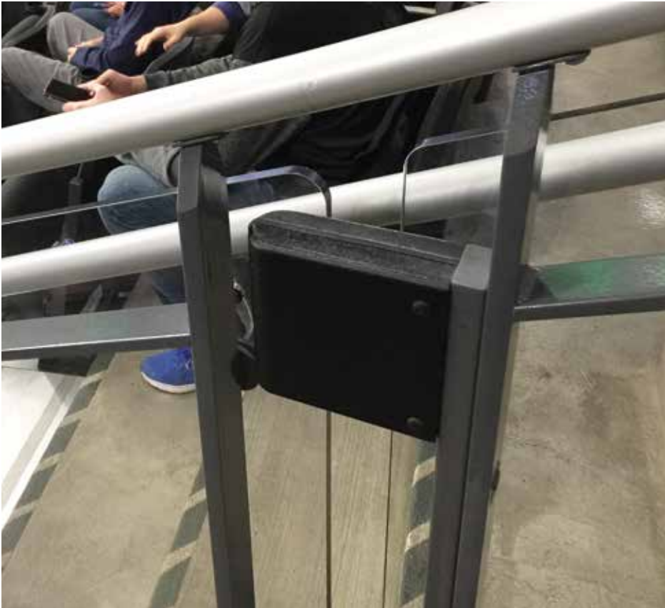
CLOCKWISE FROM LEFT: A LOWER-BOWL MINI WI-FI ENCLOSURE; A DAS ANTENNA HIDDEN ABOVE A CONCOURSE; A WI-FI ENCLOSURE CAMOUFLAGED IN A CLUB AREA.
