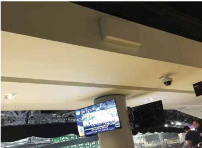
CLOCKWISE FROM TOP LEFT: A WI-FI ENCLOSURE ABOVE THE UPPER SEATING DECK; THE OUTDOOR VIEW FROM THE PANORAMA LOUNGE; MORE WIRELESS EQUIPMENT WITH A DISCREET PRESENCE.
