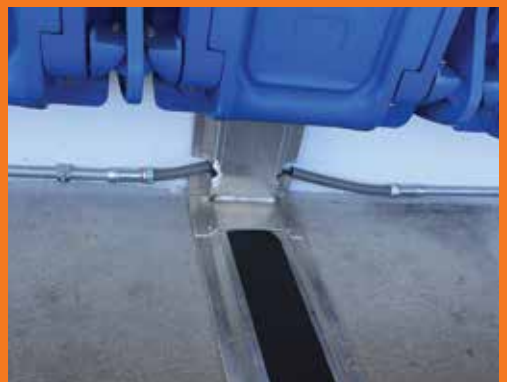
CLOCKWISE FROM TOP LEFT: WI-FI APs ARE VISIBLE UNDER BENCHES AND CLUB SEATS; A CONCOURSE DEPLOYMENT; METAL FLASHING AND CONDUITS BRING CABLES TO UNDERSEAT APs; UNDER-SEAT APs VISIBLE AS WHITE DOTS IN THE STANDS; CONDUIT UNDER THE SEATS HEADS UP IN ORDERLY FASHION; A QR CODE OFFERS A QUICK WAY TO DOWNLOAD THE APP; AND CENTER, A TOOTHY WELCOME TO THE CLUB LOUNGE.
