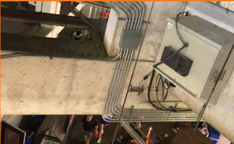
CLOCKWISE FROM TOP LEFT: WI-FI APs ARE VISIBLE UNDER BENCHES AND CLUB SEATS; A CONCOURSE DEPLOYMENT; METAL FLASHING AND CONDUITS BRING CABLES TO UNDERSEAT APs; UNDER-SEAT APs VISIBLE AS WHITE DOTS IN THE STANDS; CONDUIT UNDER THE SEATS HEADS UP IN ORDERLY FASHION; A QR CODE OFFERS A QUICK WAY TO DOWNLOAD THE APP; AND CENTER, A TOOTHY WELCOME TO THE CLUB LOUNGE.
