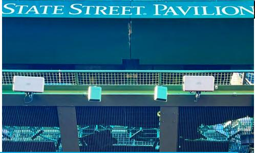
Overhangs and beams provided other mounting spots for APs covering the main seating bowl
